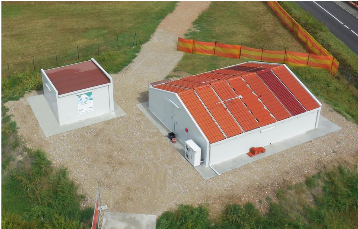
The roof tile testing site in Ferrara, Italy. Image courtesy of the University of Ferrara.
