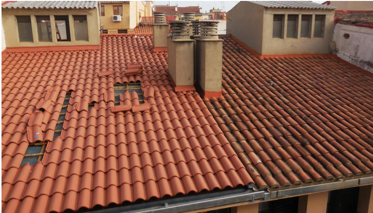
On the left, the new roof with Portuguese Herotiles; on the right, the original roof of the building in Cadelbosco with traditional Portuguese tiles
