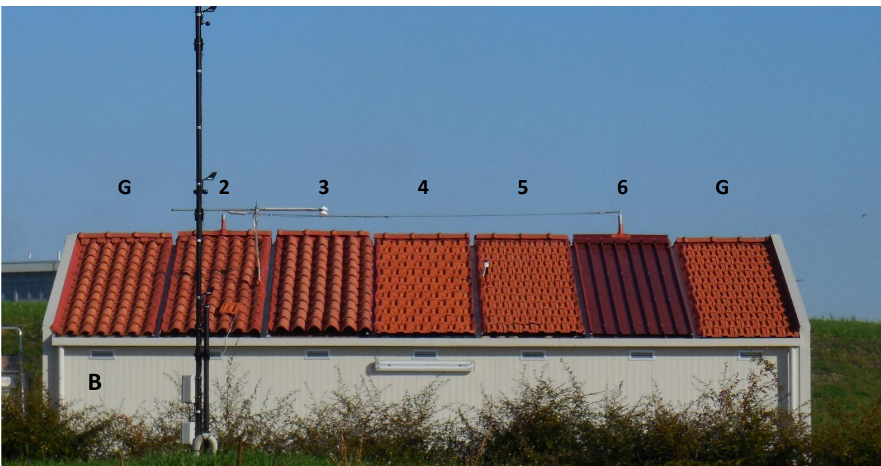
Building A: flat roof (1), located on a separate building
